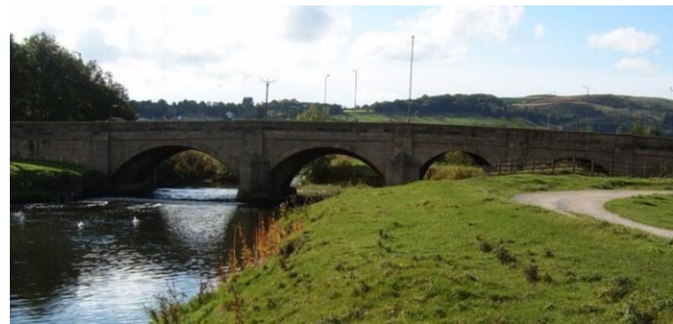
Figure 2 - Kildwick bridge photographed from the Skipton side and the Keighley side. Note the four round arches on the Keighley side, and two pointed arches and two round arches on the Skipton side.
