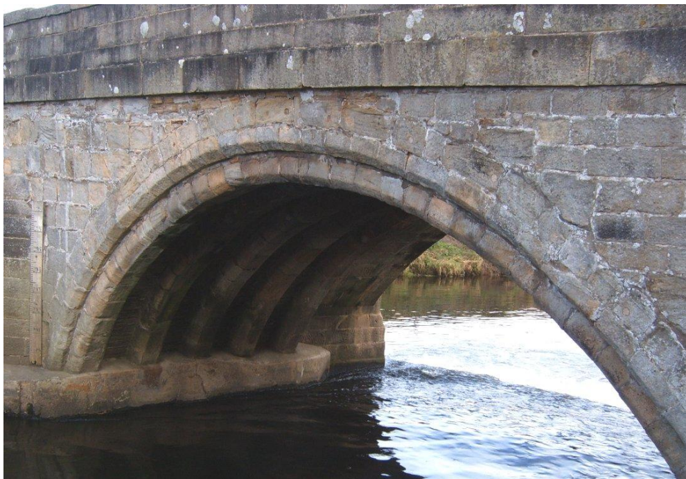
Figure 3 - Kildwick bridge photographed from the Skipton side. The two sections of the bridge can be clearly seen, with the ribbed vaulting (nearest) representing the 14 th century bridge and the plain barrel vaulting (furthest) the 1780 widening work.
