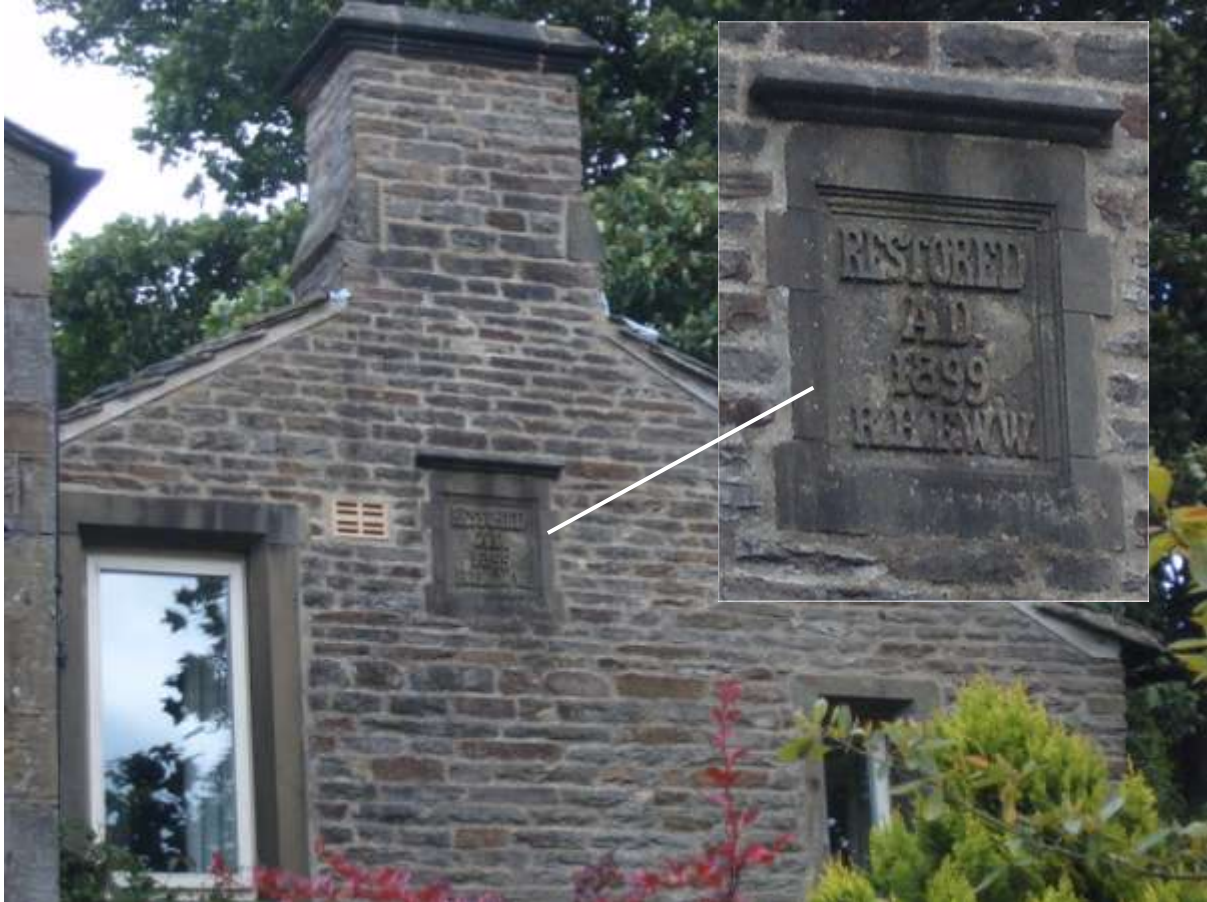
The Old Priory, at the top of Priest Bank Road – restored by Richard Francis Henry Wharton Wilson in 1899
